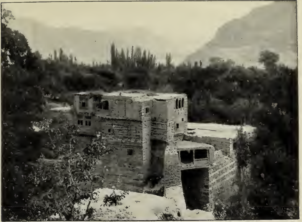
RAJAH'S HOUSE AT SHIGAR.
